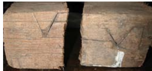
Numbered stud sections removed to level front wall to replacement sill. Colonial Williamsburg commented that the method of Roman numbering with the connected numerals was unusual. It occurs again on the fireplace wall.
