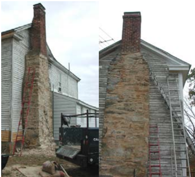
Left: East Chimney during restoration; Right: West Chimney during restoration.
