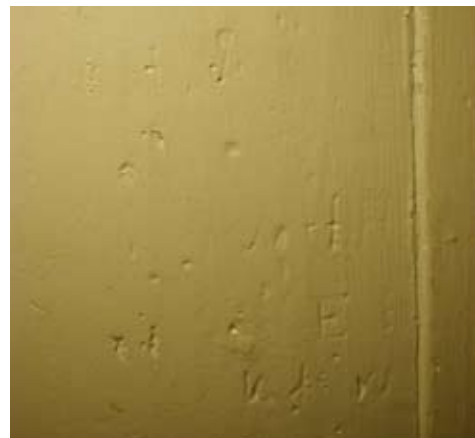
Numbered stud sections removed to level front wall to replacement sill. Colonial Williamsburg commented that the method of Roman numbering with the connected numerals was unusual. It occurs again on the fireplace wall.
